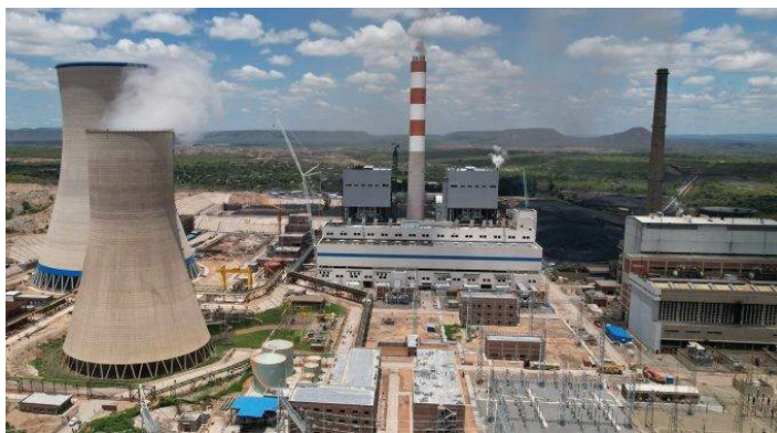
Hwange Thermal Power Station Units 7 and 8 Expansion Project
